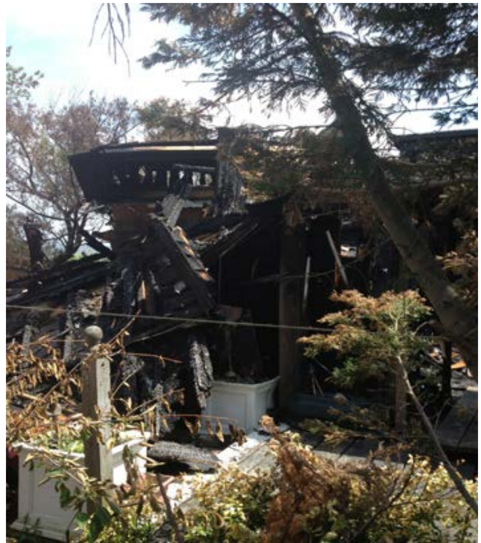
Home destroyed in Cherry Grove on 6/16 Photo credit: Nicole Brems
